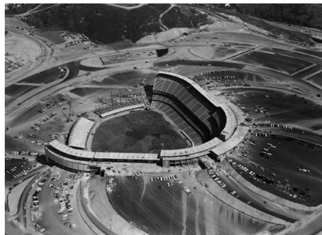
A birds-eye view of the Dodger Stadium construction and terraced parking at Chavez Ravine.
